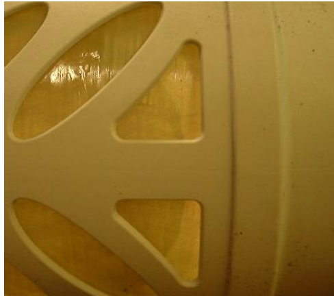
Figure 3b — Delamination and no surface damage - acceptable
