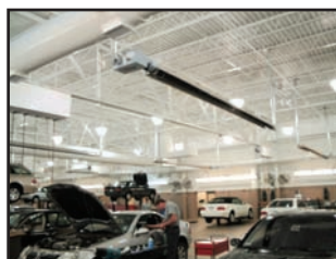
Vehicle Maintenance Facilities
